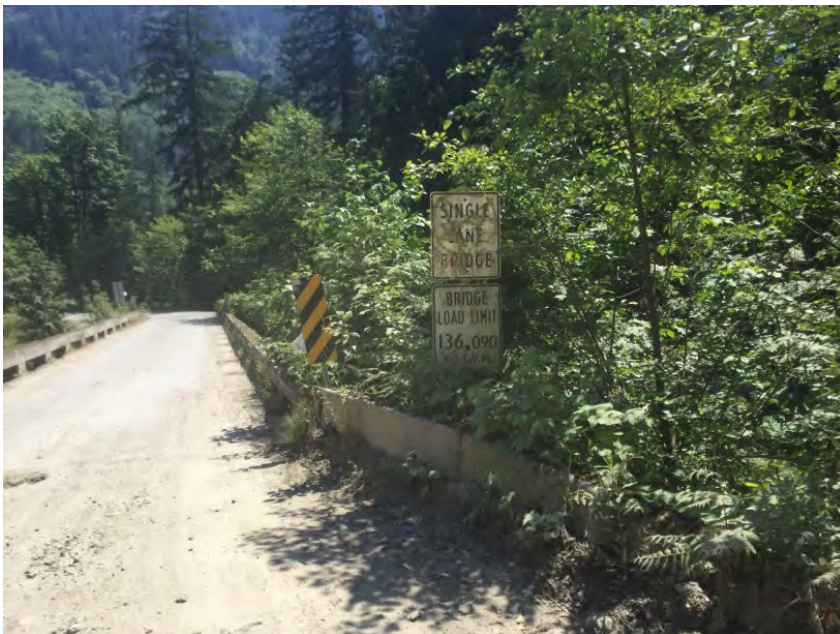
Load Rating Sign
