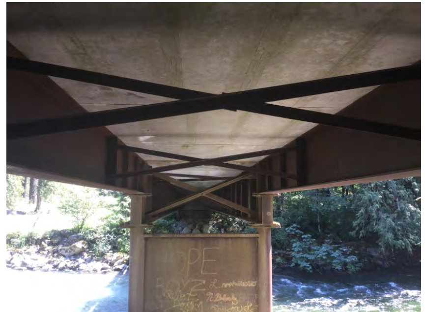
Jump span superstructure
