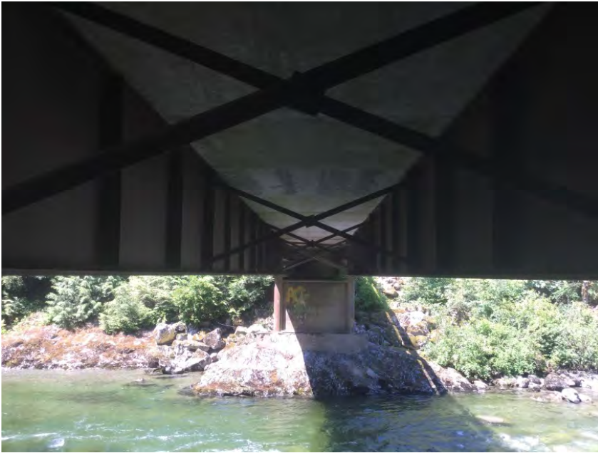
Main span superstructure
