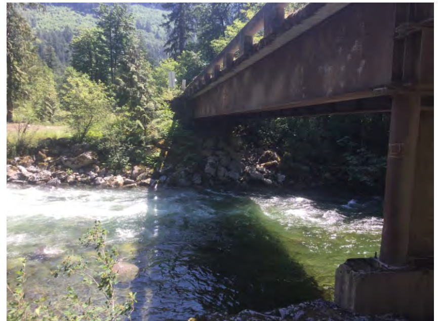
Left Bank Abutment when facing downstream
